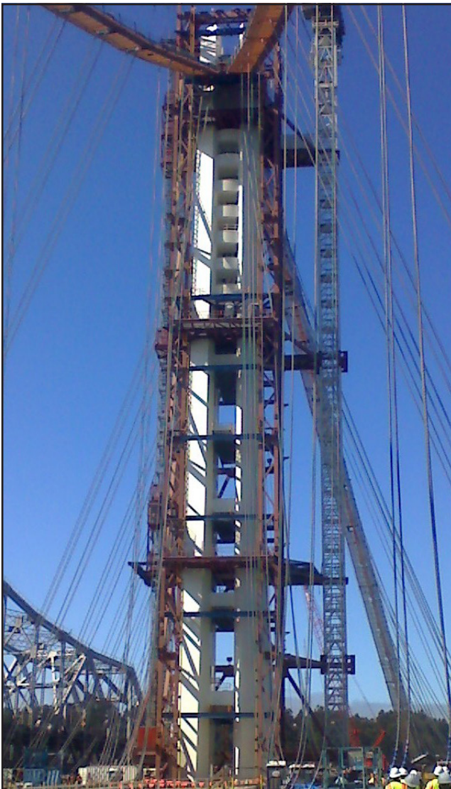
Closeup of the San Francisco / Oakland Bay Bridge Tower
