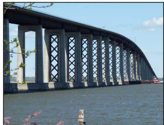
Antioch Bridge Seismic Retrofit
