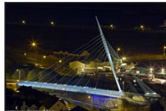
Fabian Way Cable-Stayed Bridge - UK
