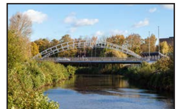
Taunton Third Way Bridge - UK
