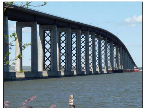
Antioch Bridge Seismic Retrofit
